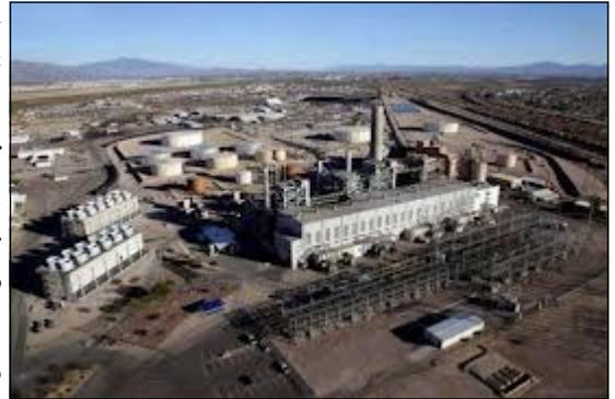
At the H. Wilson Sundt Generating Station, power is generated by two gas turbines and four steam turbines ranging from 83 to 165 megawatts. The steam units can be fueled by coal, natural gas, or fuel oil. In addition, landfill gas from Los Reales landfill is used. Generally, though, about 90% of the power generated at the station is from coal.
